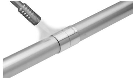
5. Allow the solder to come into contact with the joint as the propane torch heats the opposite end to where the solder is being applied. Apply solder all around the joint. Solder should liquify when it comes in contact with the fitting and flow into the joint.
