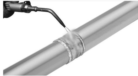
5. Allow the brazing alloy to come into contact with the joint as the propane torch heats the opposite end to where the alloy is being applied. Apply alloy all around the joint. Solder should melt when it comes in contact with the fitting and flow into the joint.
