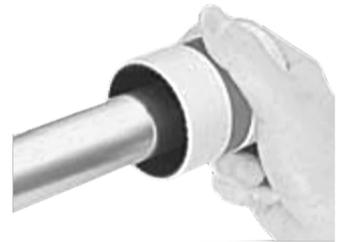
4. Clean the outside of the pipe using steel wool (or 120 grit emery cloth).
