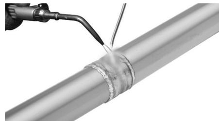
6. Inspect joints to ensure brazing alloy is covering the full joint and there is no no areas for potential leakage. Allow to cool and wipe off any excess flux if necessary. Flush out the pipework.
