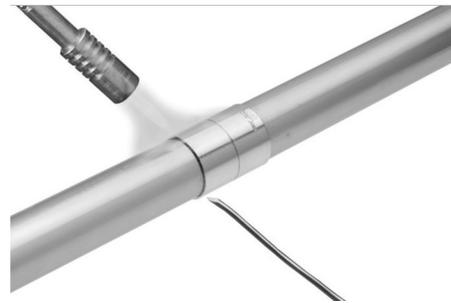
6. Inspect joints to ensure solder is covering the full joint and there is no areas for potential leakage. Allow to cool and wipe off any excess flux. Flush out the pipework.
